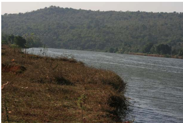
Unprotected Bank of estuary at Kondsar
