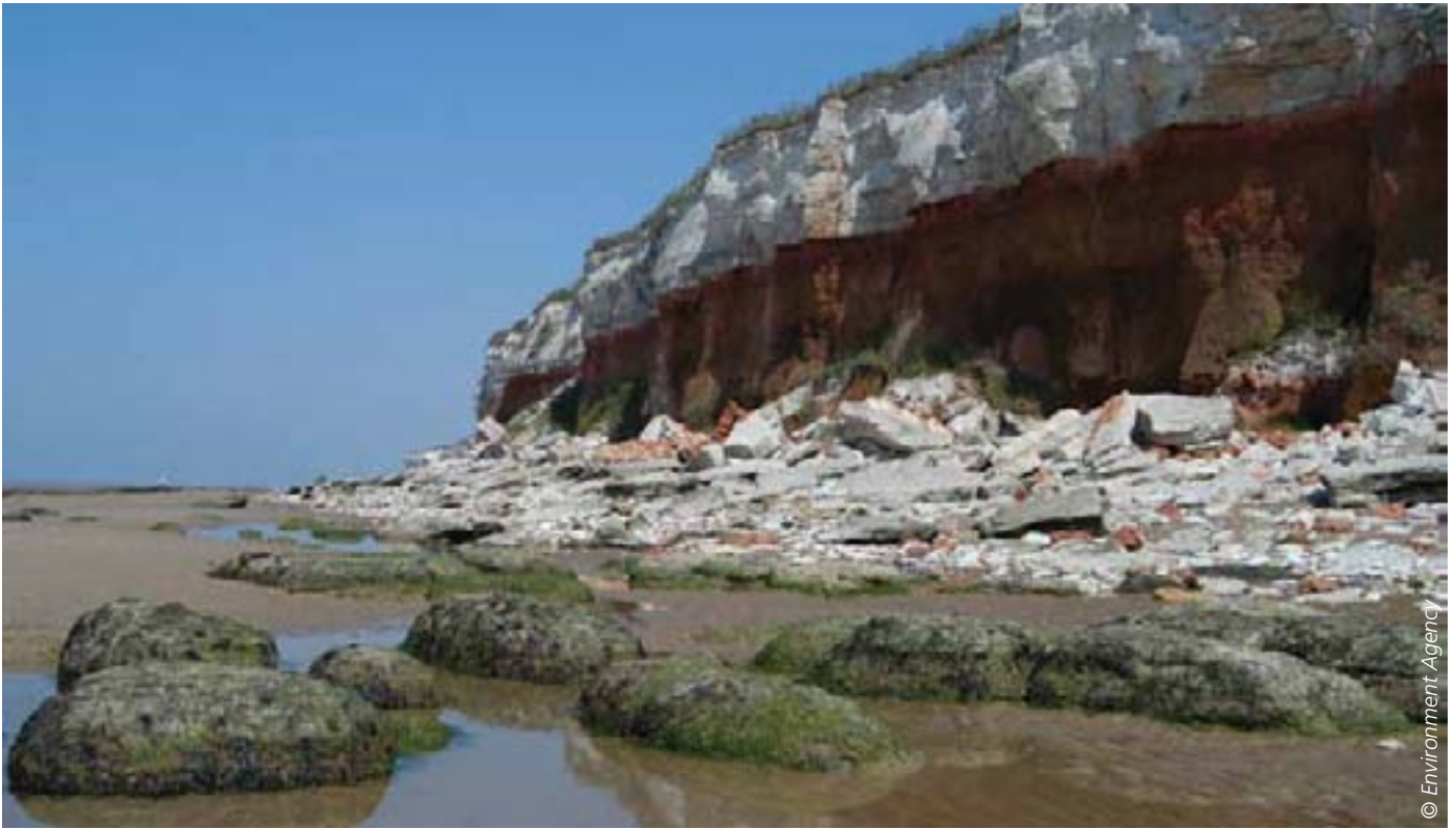
Erosion at Hunstanton cliffs, Norfolk. Rising sea levels are affecting a large proportion of the coast in this region
